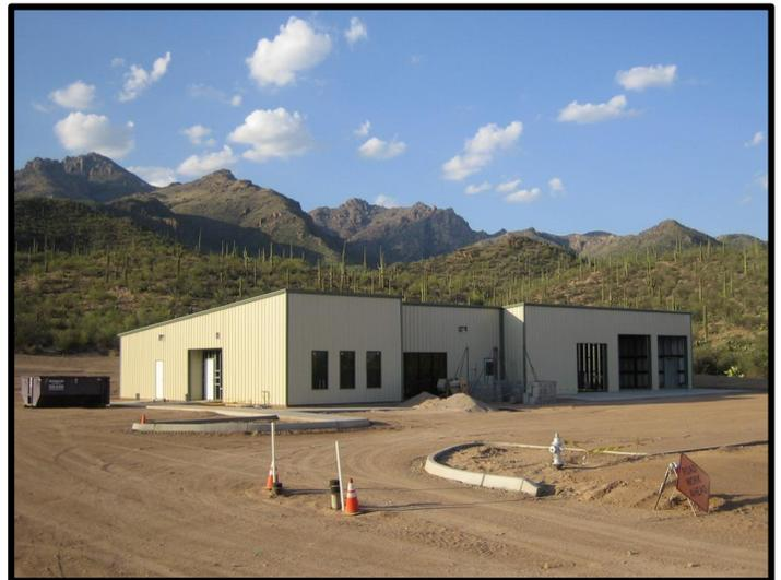
Construction continues on the Sabino house. Currently the shell is completed and doors and windows are up. Electrical and plumbing are in progress. We are still looking for in kind or monetary donations. Some projects can be completed by SARA members willing to donate time and labor; contact Rich Kunz if you have any questions.
